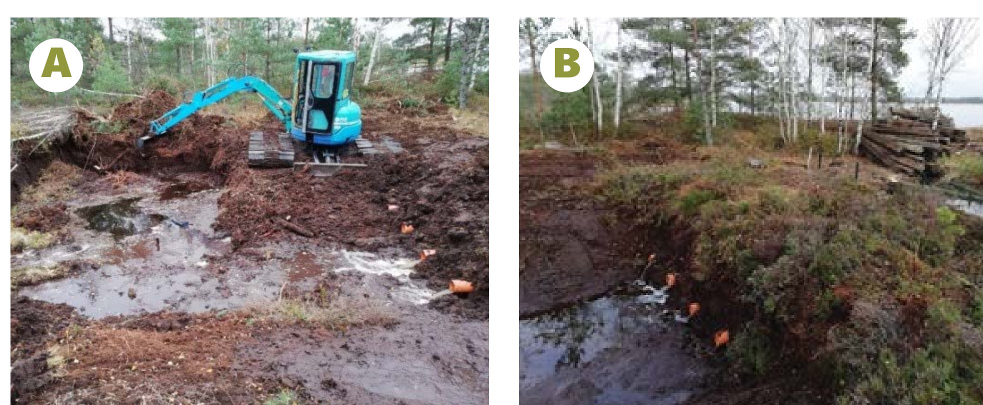
Figure 4. A - Peat dam construction. B - The same peat dam when construction is complete. Photo: Juris Pētersons
